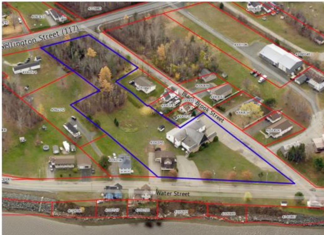
Figure 2: Oblique Aerial Image of Subject Properties outlined in blue
